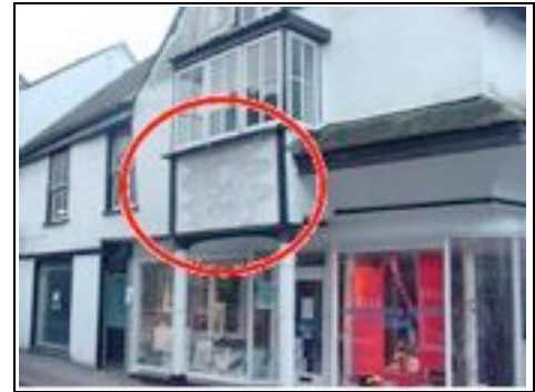
Deteriorating render
