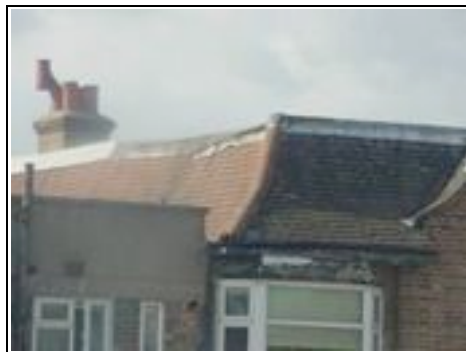
Mansard roof with hidden flat roof
