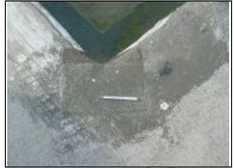
Example of patch repair
