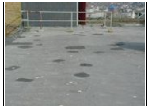
Patch repairs looking towards the rear of the property
