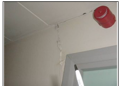
Cracking to right side
