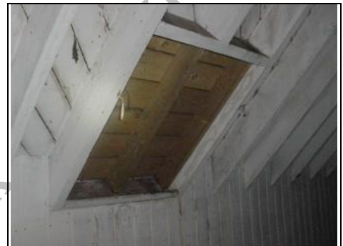
Blocked up roof window
