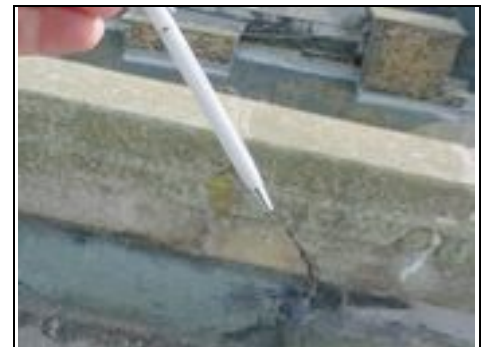
Cracking to parapet
