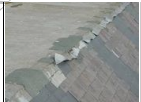
Old repairs lifting
