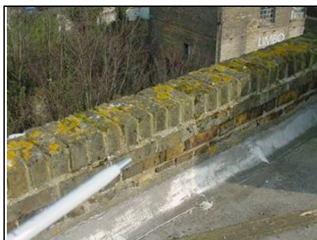
Moss on rear parapet wall indicating that dampness is getting in
